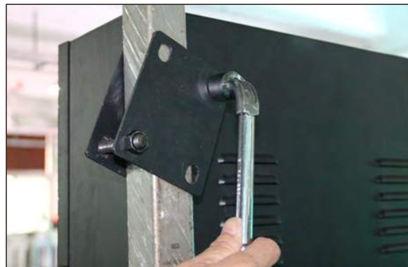
Step 3: Fix the screws and adjust the uniformity and gap
